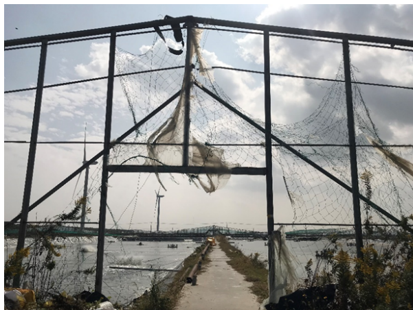
(Plastic shed blown by the typhoon in the California perch outdoor fish fry farm)
